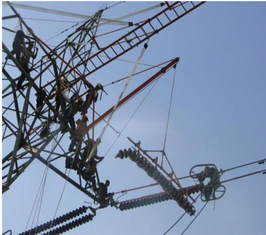
Fig.14 insulator string replacement on 400KV line [10].
