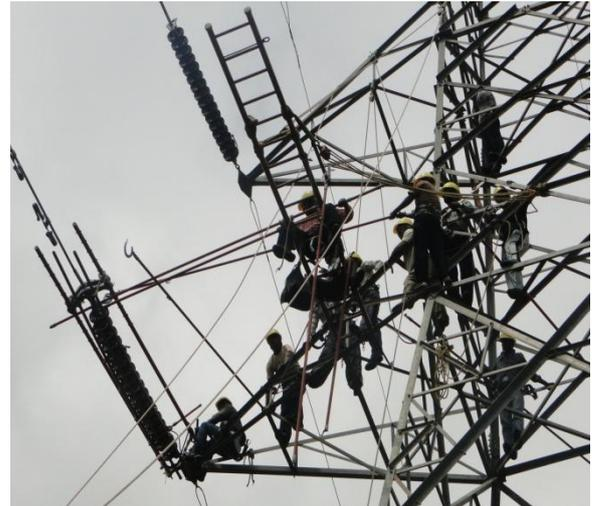
Fig.12: Changing of insulators on 220 KV Dead End [10].
