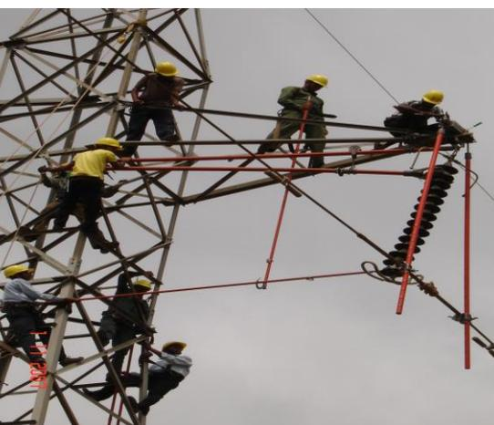
Fig.10: Changing of insulator on 220 KV Suspension Point [10].
