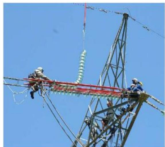
Fig.13 Changing of insulator string on 400 KV Dead End [10].
